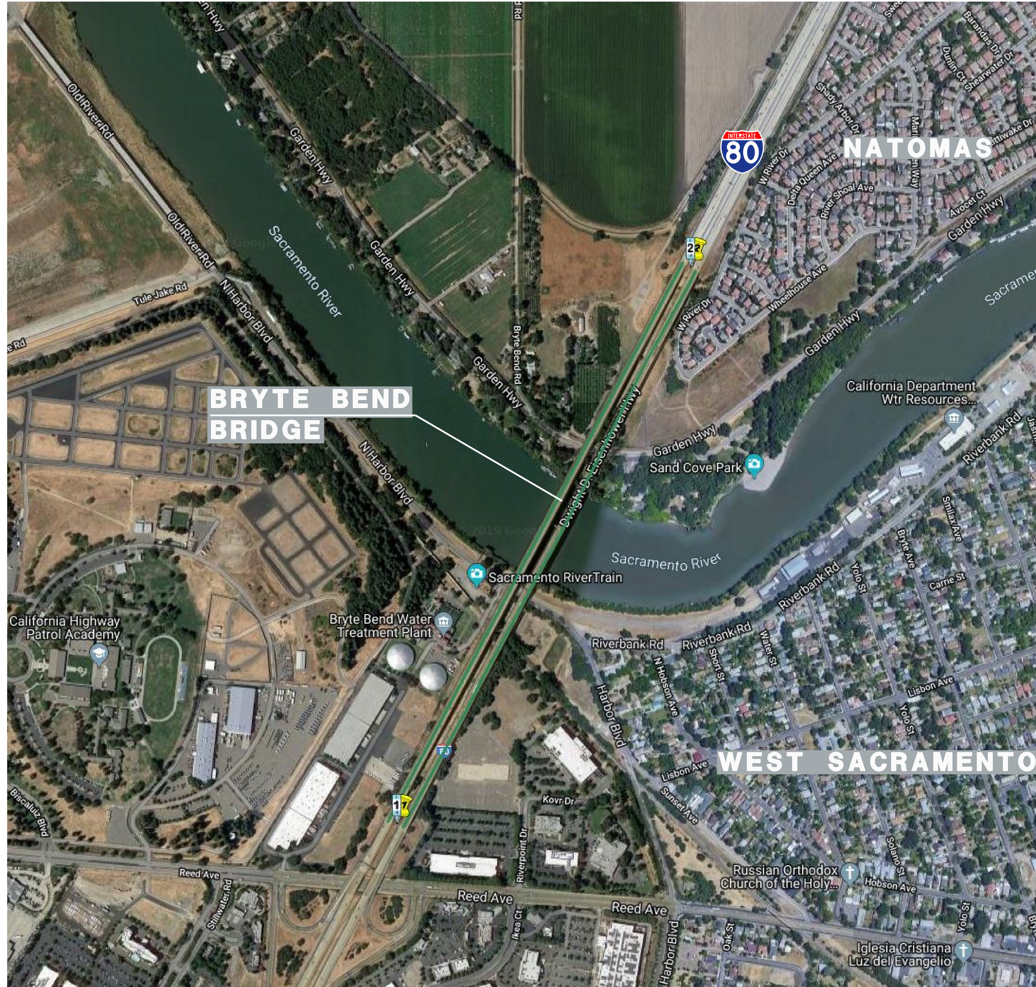
SACRAMENTO RIVER BOH (BRYTE BEND BRIDGE)
