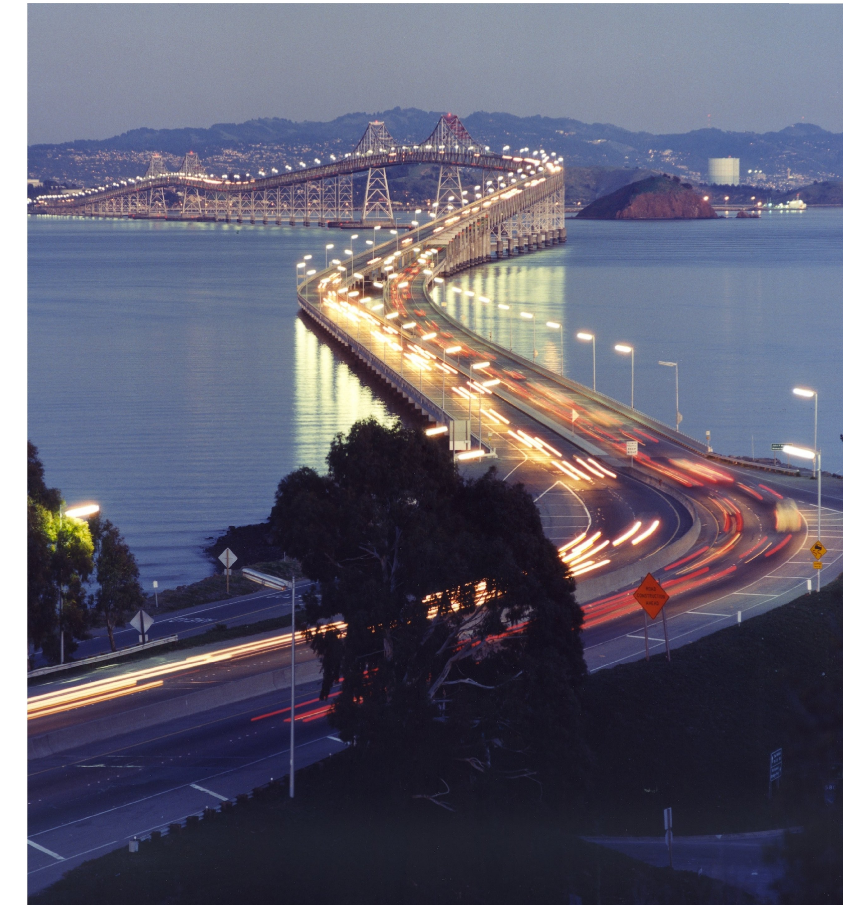
BRIDGE DECK LIGHTING EXAMPLE RICHMOND-SAN RAFAEL BRIDGE - METROPOLITAN TRANSPORTATION COMMISSION
