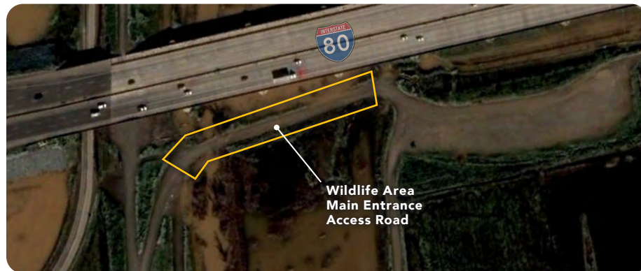
Wildlife Area Main Entrance subject to routine nuisance flooding that limits public access.
