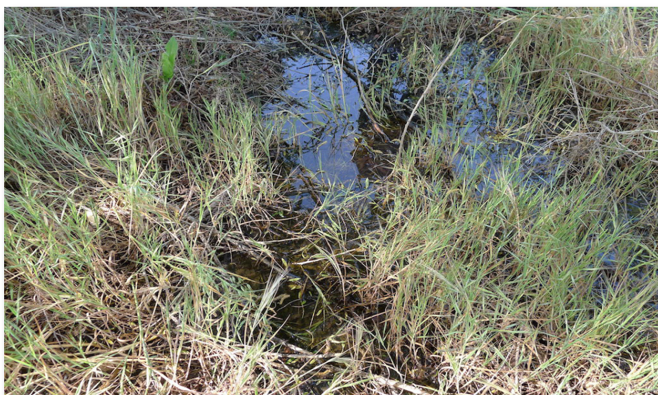
Photo 6. Leakage flow ponded at the toe of slope, on April 24, 2018. Grass is Cynodon dactylon (FACU). If surface water such as this had been present throughout the winter, vegetation would be dominated by FAC or wetter species. Instead, this is fresh leakage flow, with the irrigation system just having been activated as the weather warms up. DP-2 is located within a few feet of the standing water visible here.
