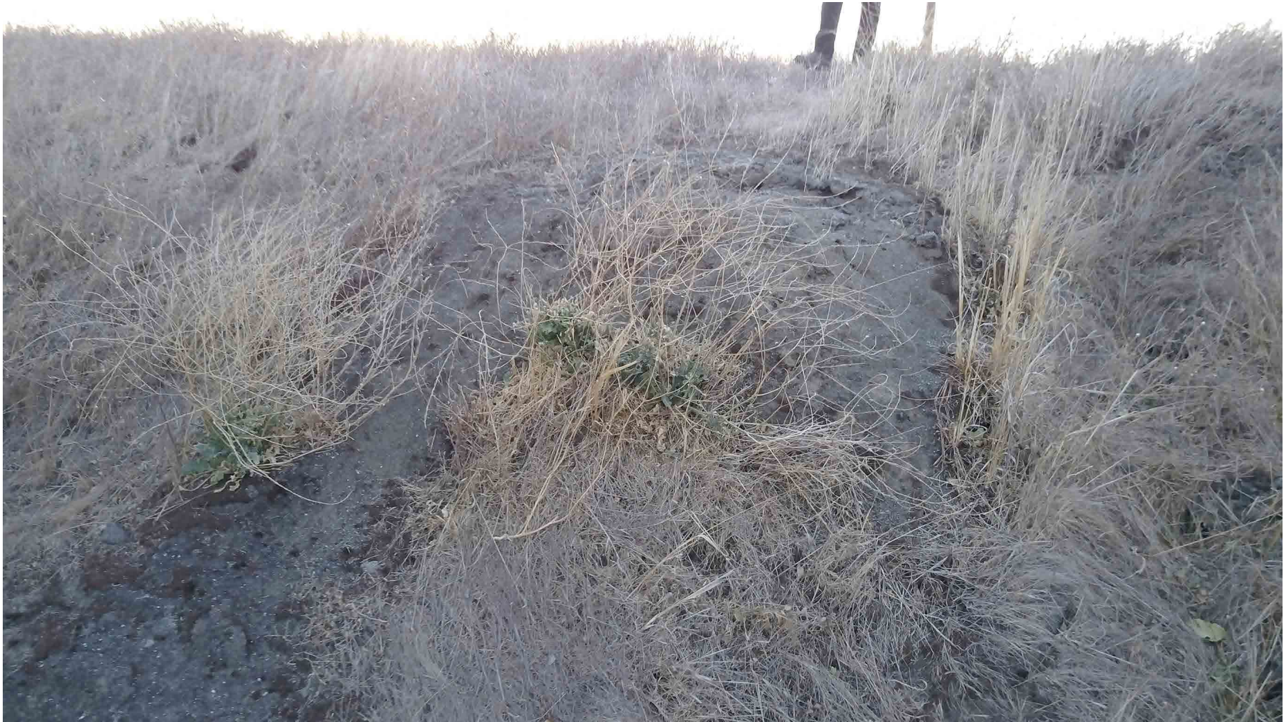
Photo No. 4 Asphalt concrete armoring on upper bank
