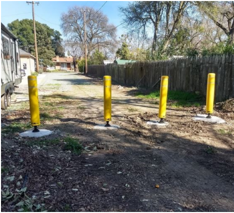
Pedestrian and traffic safety improvements at Poplar St. in Clarksburg.
