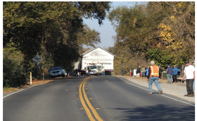
Re-location of the 1893 Clarksburg Schoolhouse.
