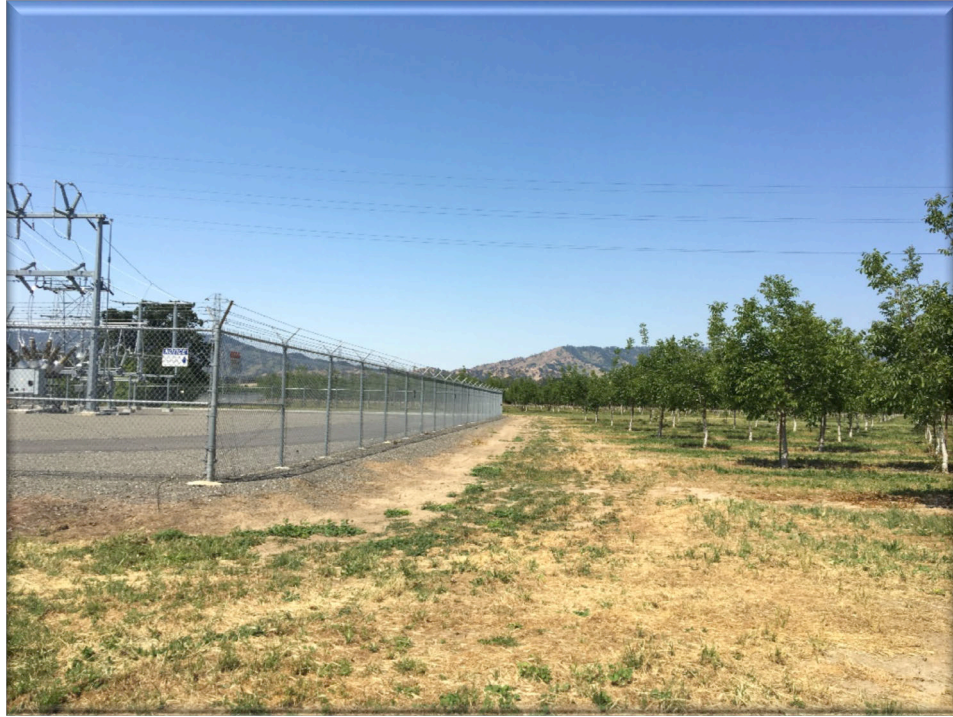
Plate 15. Looking west along the northern border of the substation on May 9. Grassy edges adjacent to orchards and the substation are occupied by ground squirrels, but provide very marginal habitat for burrowing owls due to the overall land use and lack of larger open grasslands.
