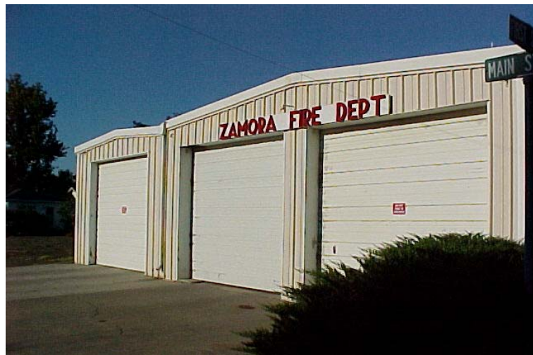
Zamora FPD Hangar Bays
