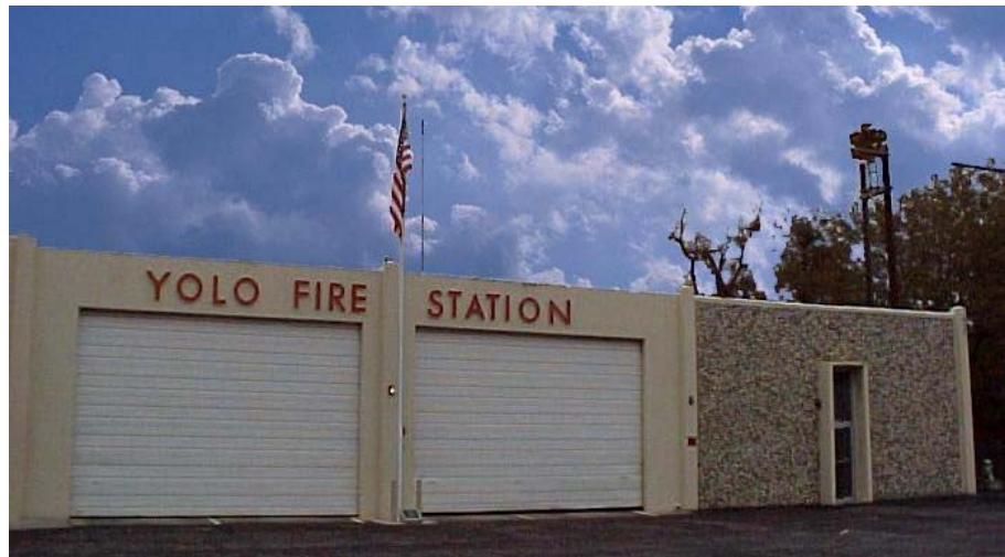
Yolo FPD Fire Station
