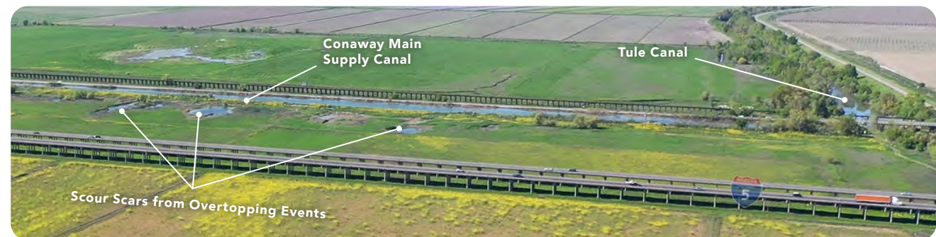
View of Conaway Main Supply Canal, looking north. Photo by Conaway Ranch.
