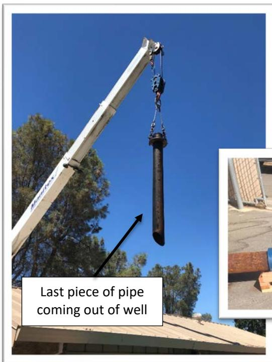
A new pump has been installed at the Canvas Back well that is able to pump water from a lower depth into the community water system. The new pump will enable the community to use the 75 feet of water remaining in the well. The pump is set at the bottom of the well and so it cannot be
