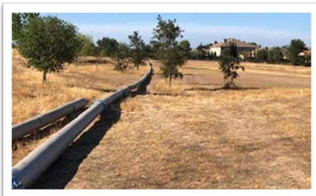
as a back-up well for the community and to irrigate the golf course. The golf course is now being irrigated from water obtained from underflow (groundwater) from Cache Creek. The water from the creek is being delivered to the golf course's irrigation pump system located at the water treatment plant through about 4,000 feet of temporary pipeline.
