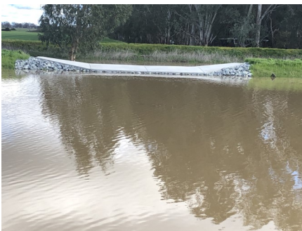
Airport Drainage Basin
