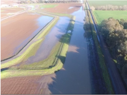
Airport Drainage Basin
