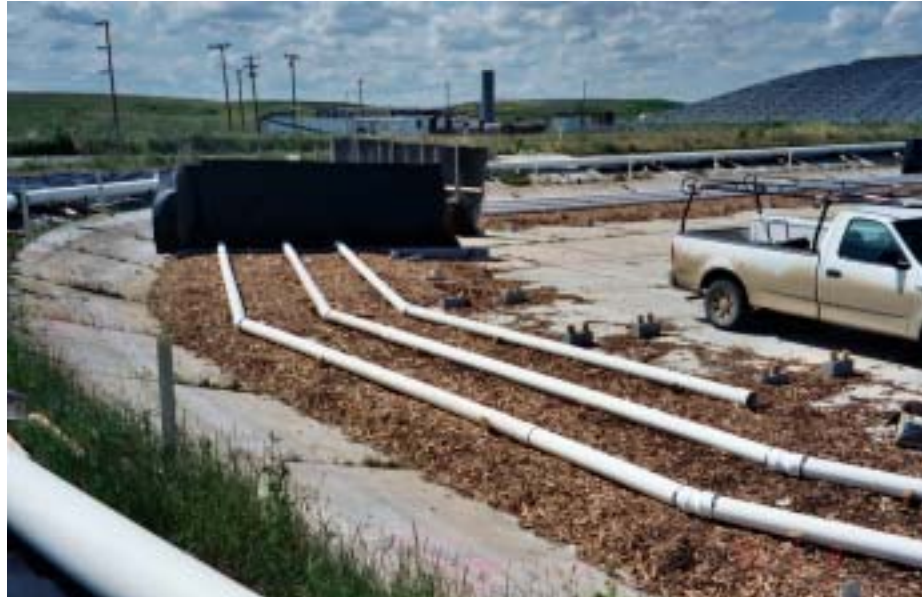
Image 5-7. Construction of the biofilter
