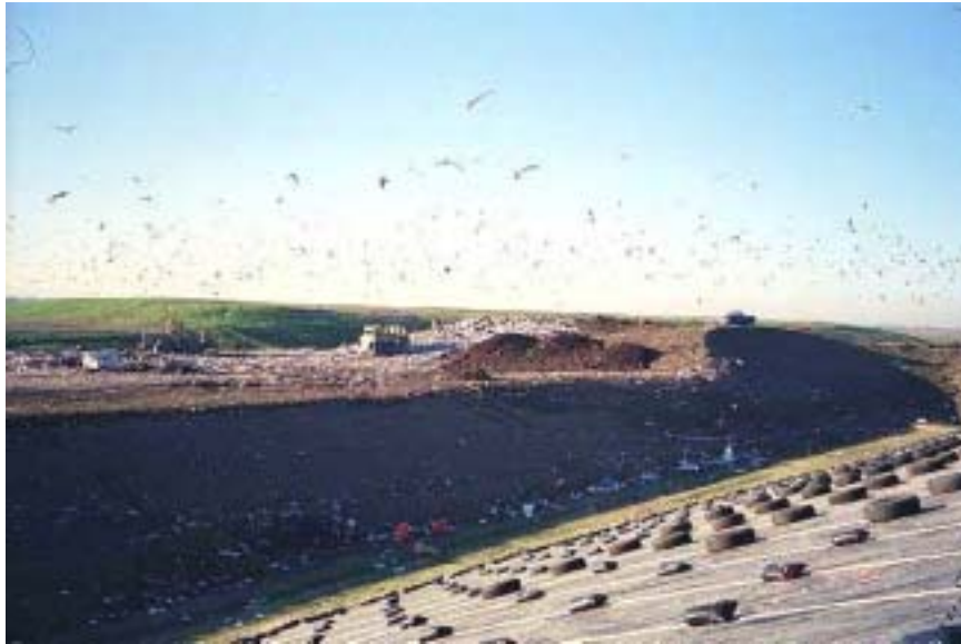
Image 4-1. Waste placement in the west-side cell
