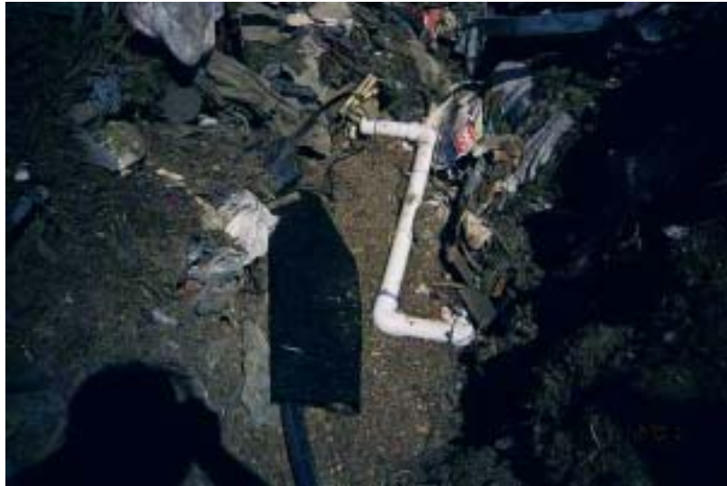
Image 3-4. Moisture, temperature , and tube installation
