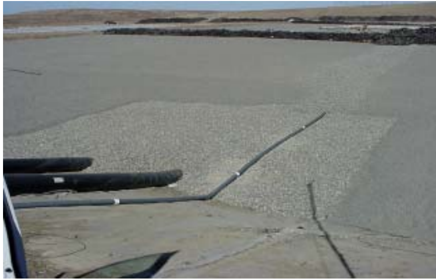
Image 3-5. Gravel drainage layer and leachate collection sump
