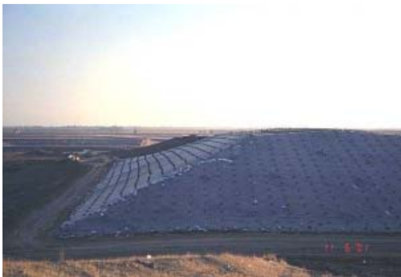
Image 3-3. Northeast anaerobic surface liner
