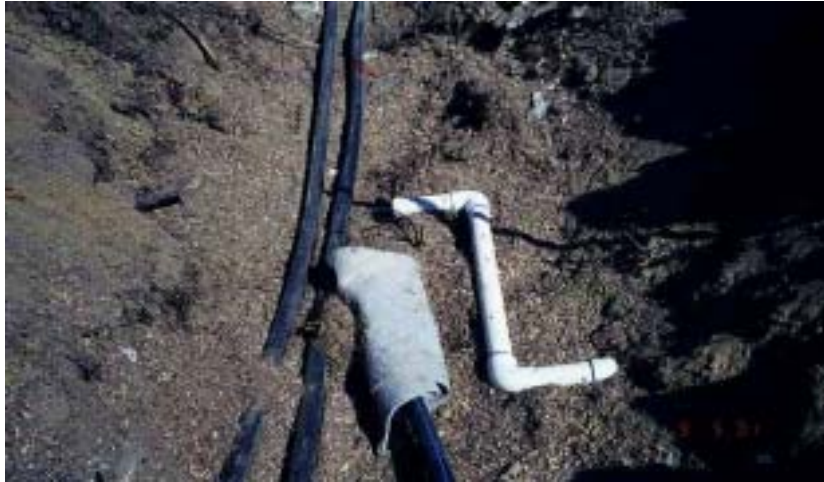
Image 5-3. Moisture, temperature, and tube installation
