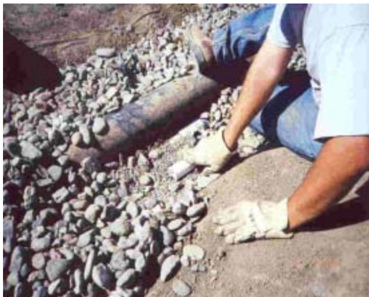
Image 6-2. Pressure tubes installed in LCRS trench
