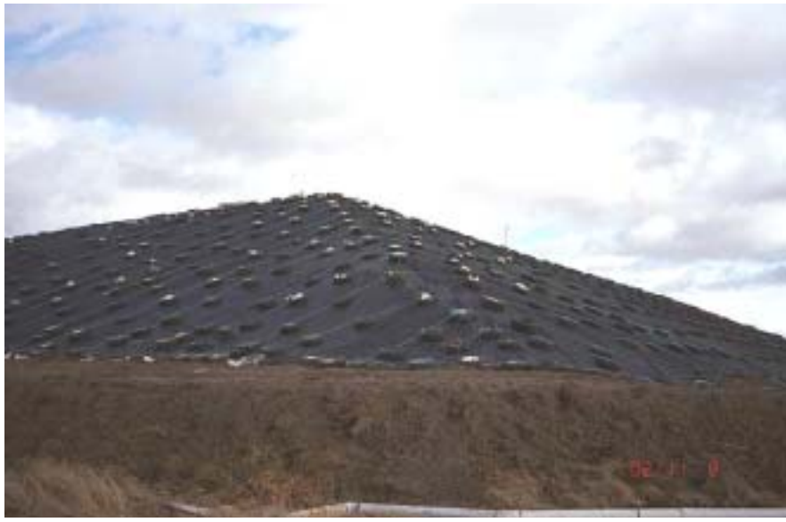
Image 4-4. West-side anaerobic cell surface liner.
