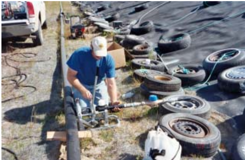
Image 4-2. Installation of valve and flow meter assembly on leachate injection lines
