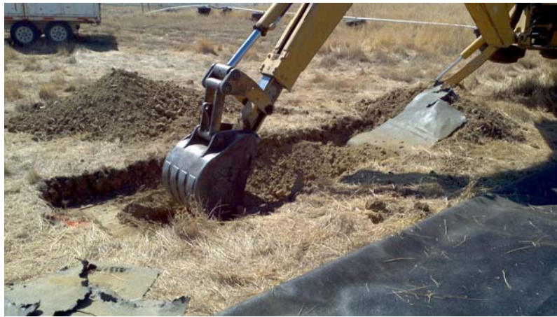
Figure 4: Excavation of cover soil below liner.
