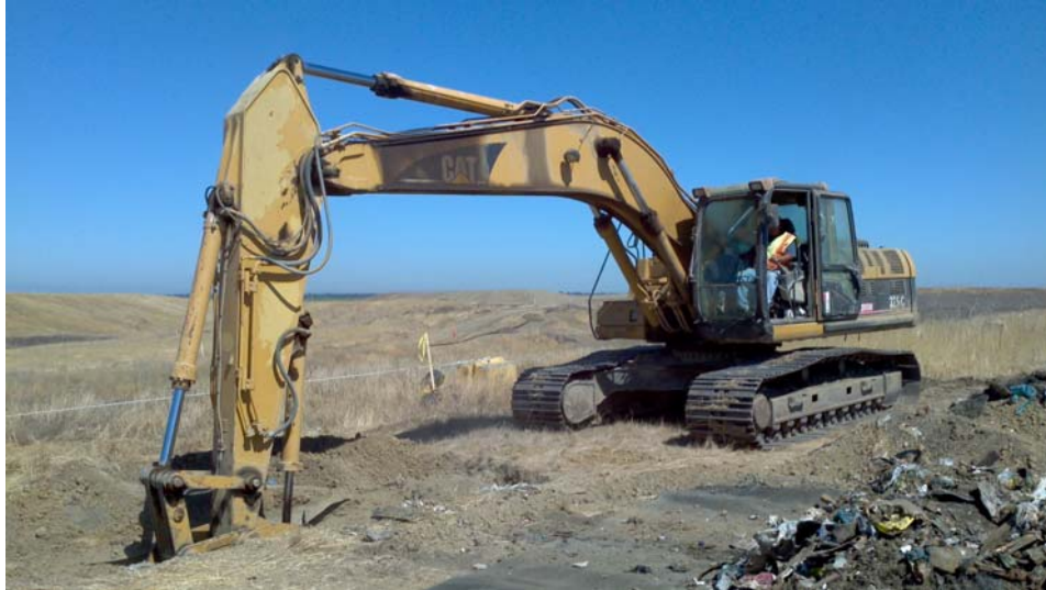
Figure 5: Excavation of waste below cover soil.
