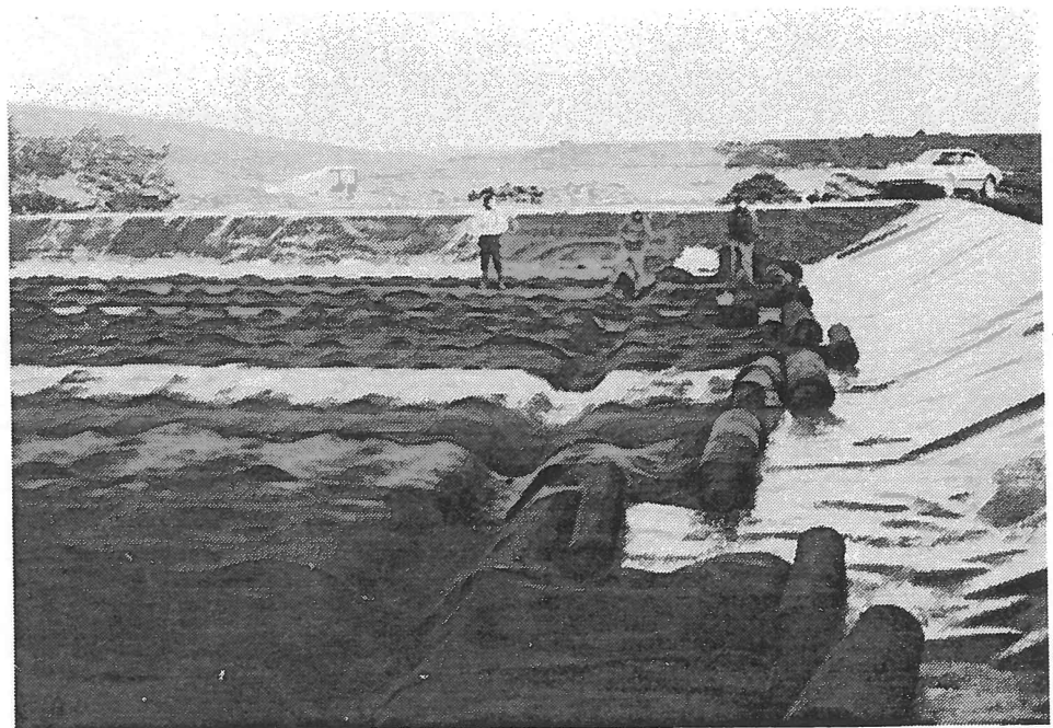
Photo 1. Placement of Geonet on the Base Liner
