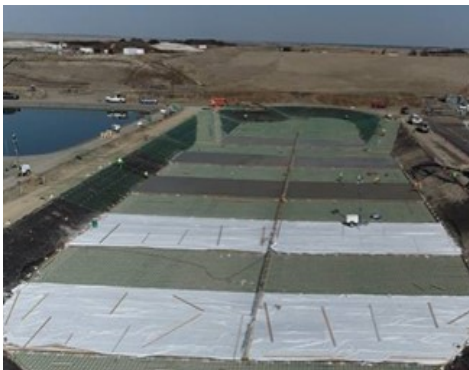
Liquid Waste Pond Reconstruction
