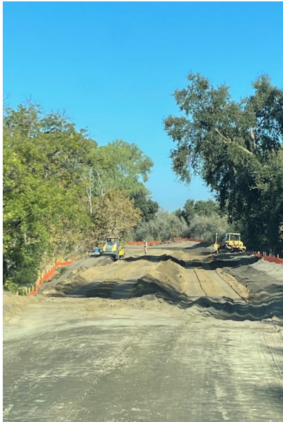
Knights Landing Levee Degrade
