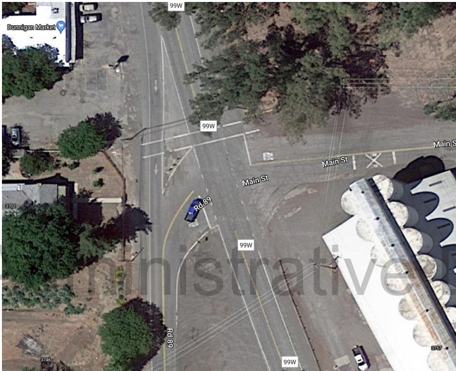
Figure 13. Main Street, CR 99W, CR 89 Intersection
