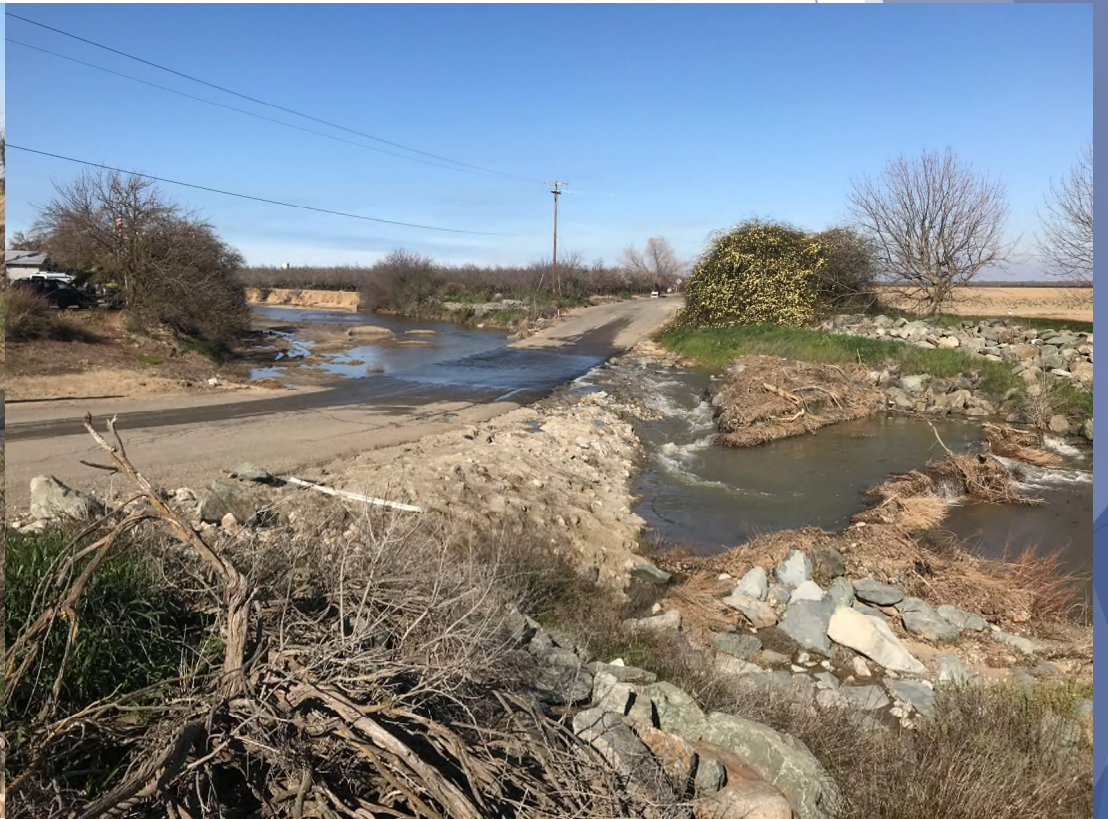
County Road 88 Crossing
