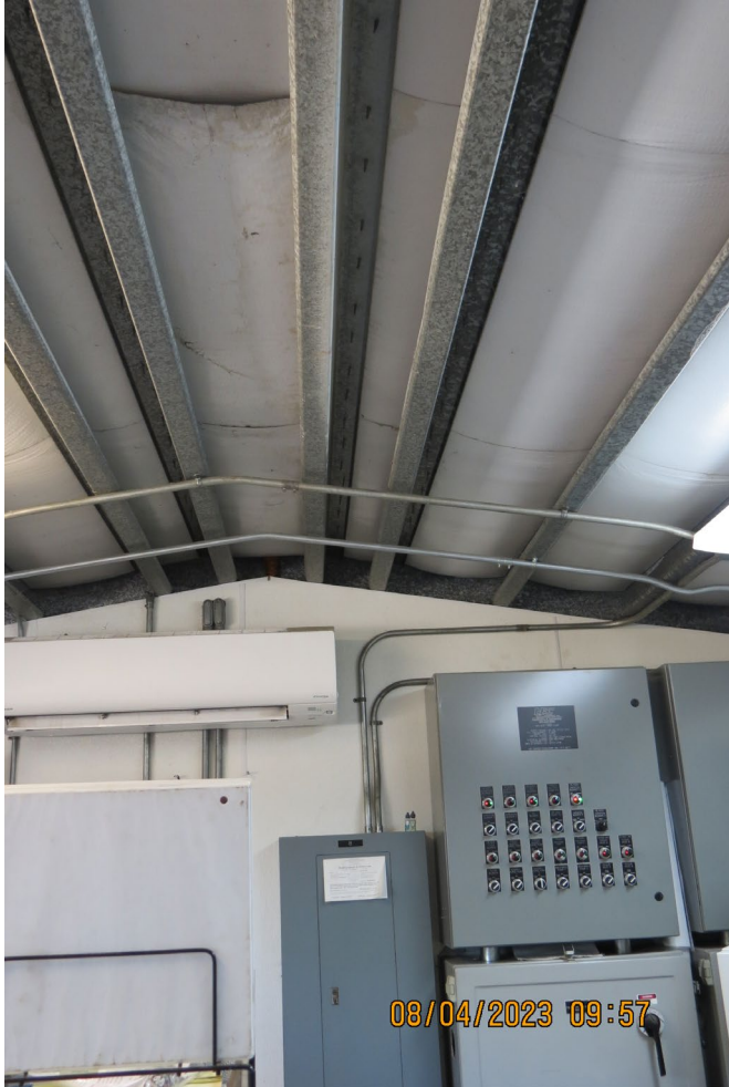
Leaky Roof Repair
