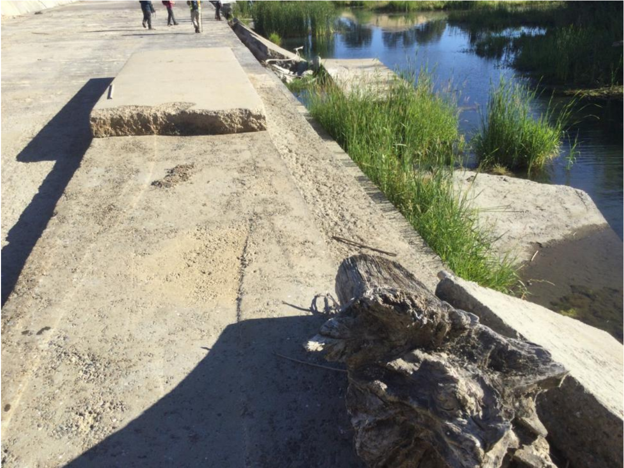
Figure 2-13. Capay Dam and apron. (2023)
