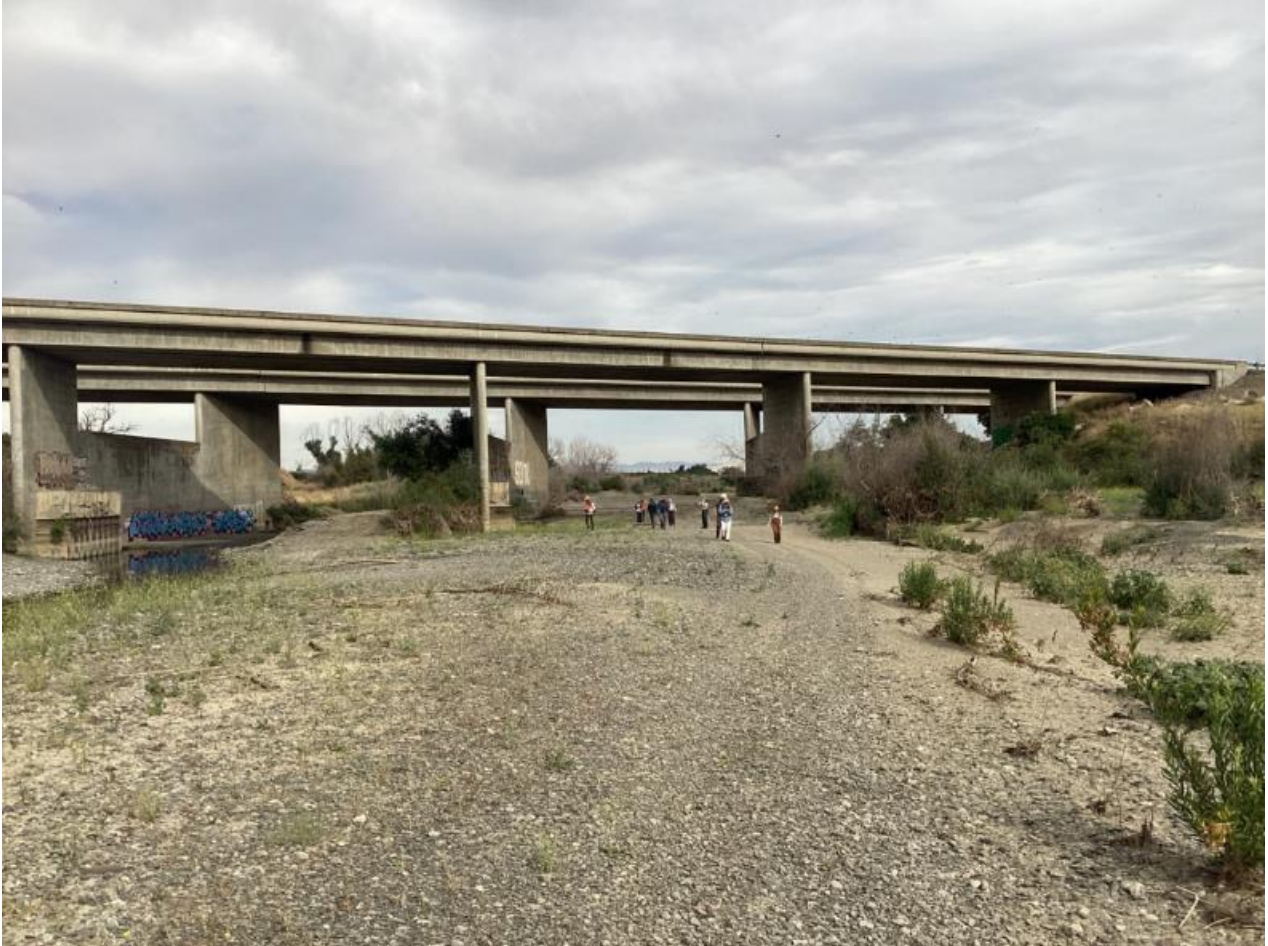
Figure 2-23. Photo showing I-505 Bridge piers. (2023)
