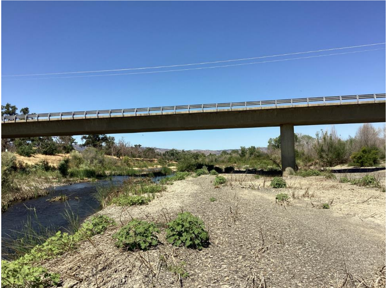
Figure 2-16. Photo showing Capay Bridge and limited vegetation growth after elevated flows from January and March. (2023)
