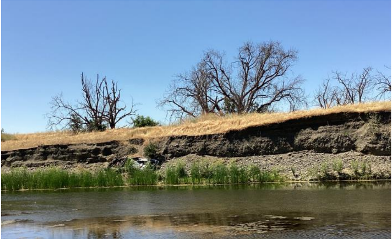
Figure 2-17. Photo showing car in the streambank at RM 25.9. (2023)
