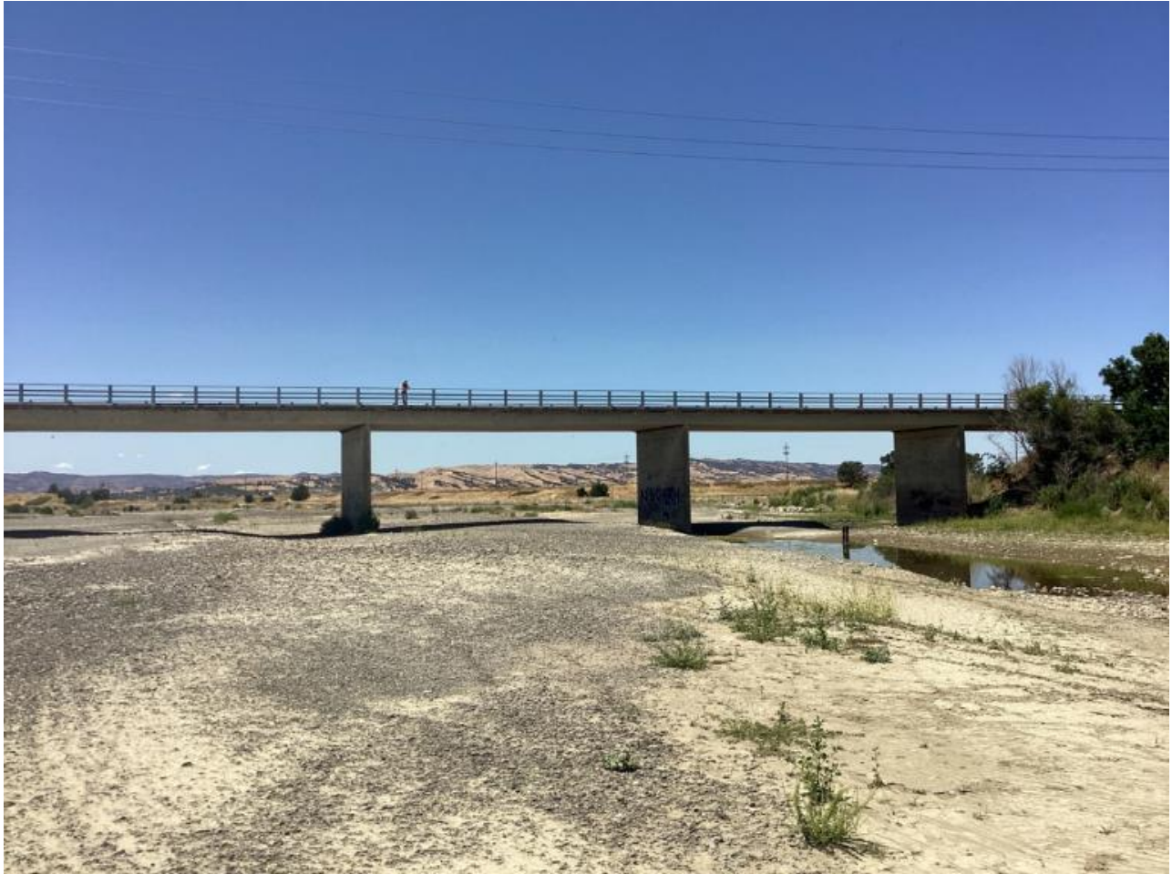
Figure 2-21. Esparto Bridge Piers with no significant change from last year. (2023)
