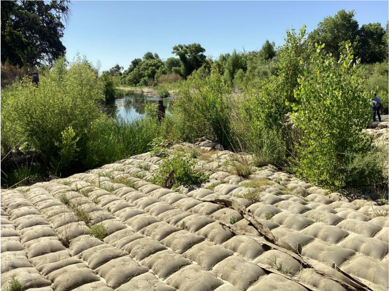
Figure 2-15. Current state of erosion control blanket at PG&E Palisades site. (2023)
