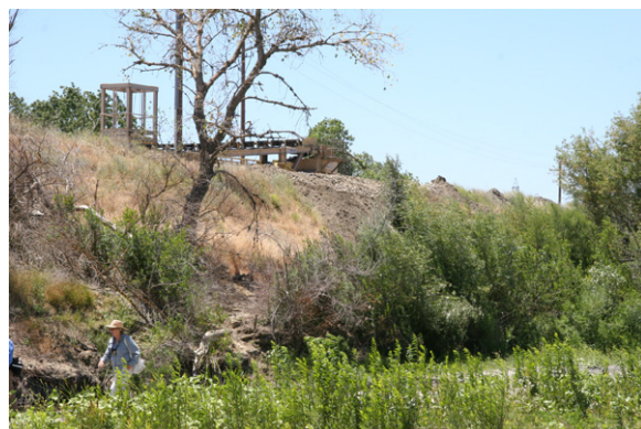
Figure 51: Gravel spill below conveyor transfer site at RM 19.7.
