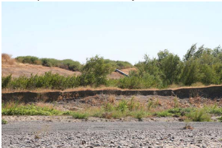
Figure 40. Drainage pipe has outflow onto a low terrace surface contained within the main channel.
