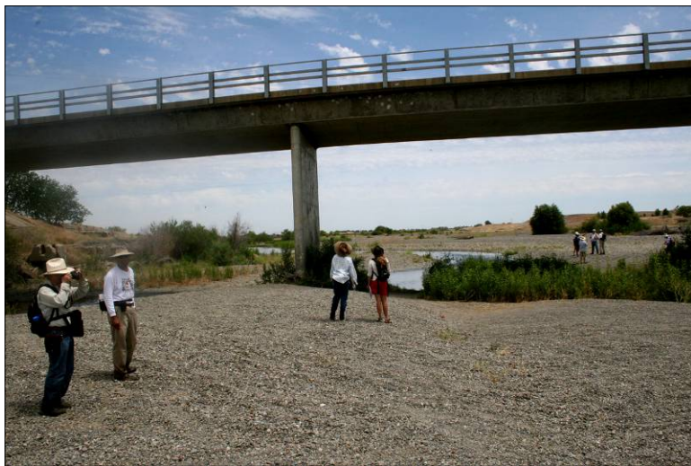
Figure 27. The CR-87 Esparto Bridge abutments.
