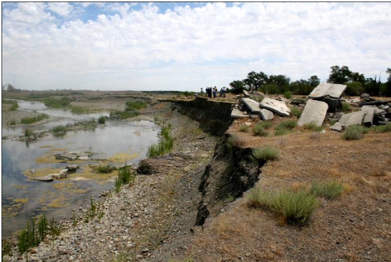
Figure 22 (above) and 23 (below). Creek meander eroding bank and concrete posed to fall into the Creek.
