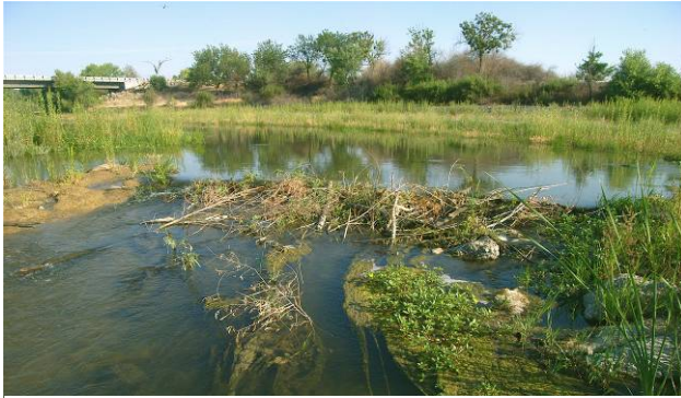
Figure 17: Beaver dam downstream from CR-85 Capay Bridge.
