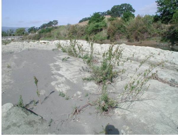
Figure 4. Seeps at the base of the soil profile in the Capay Sub-Reach caused by irrigation and drainage from the West Adams Canal.
