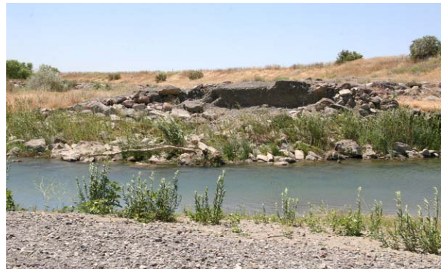
Figure 43: Erosion at upstream (south bank) spur dike, RM 21.3 in 2007 (left) and 2008 (right).
