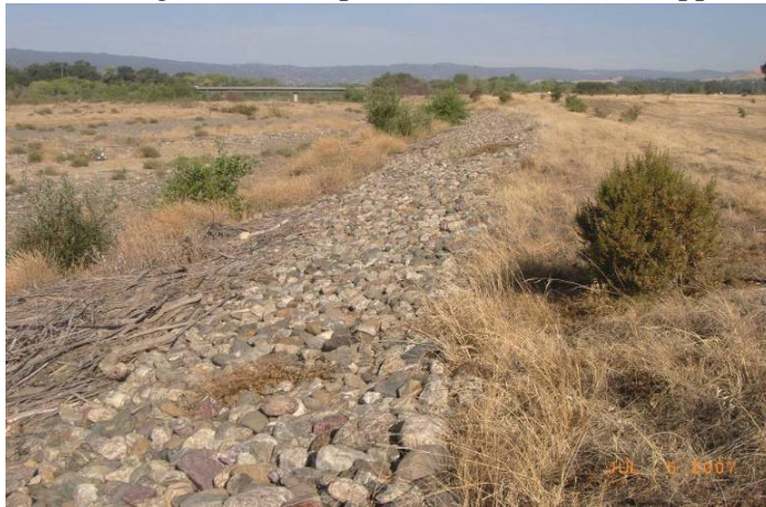
Figure 20. Bank protection extending downstream of Capay Bridge
