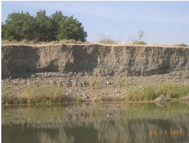
Figure 21. Craig Property eroding bank due to Creek meander.
