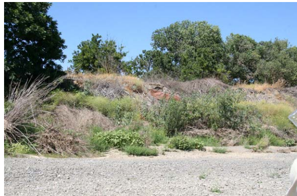
Figure 63. Crushed car stabilizes the bank at RM 17.8.
