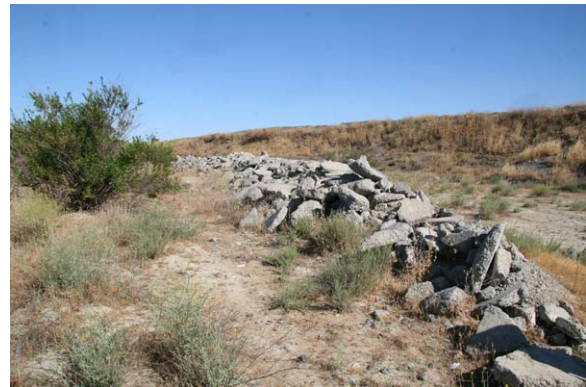
Figure 36: Bare concrete rubble protects the base of the levee at RM 23.2.
