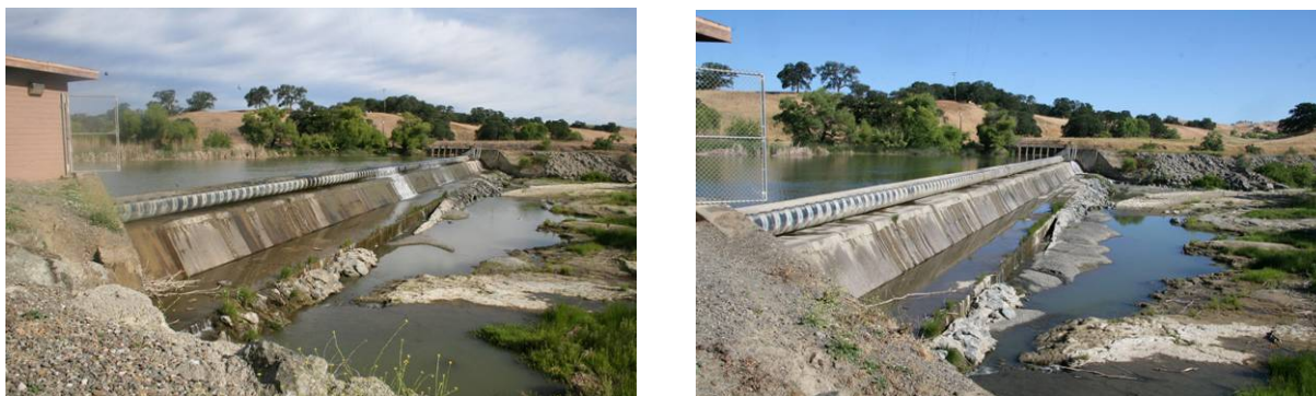
Figure 6. 2007 photo of Capay diversion dam.
