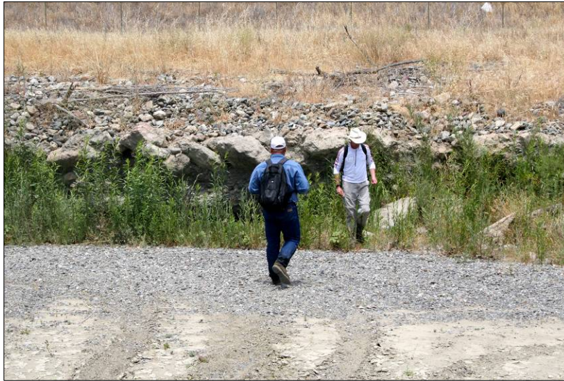
Figure 24 (above), 25 (below left), and 26 (below right). Granite Co. bank stabilization eroding at the toe.
