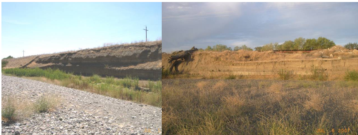
Figure 55. Location for proposed bank stabilization by CEMEX approved by the TAC in 2007.
