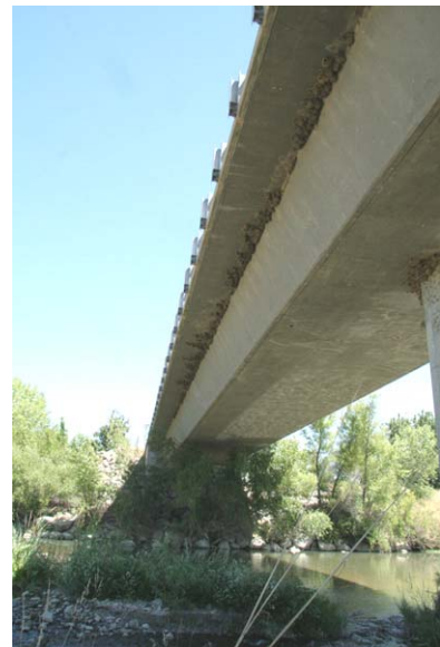
Figure 16: Cliff swallows under CR-85 Capay Bridge.
