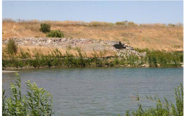
Figure 44: Erosion at second downstream spur dike (south bank), RM 21.25.
