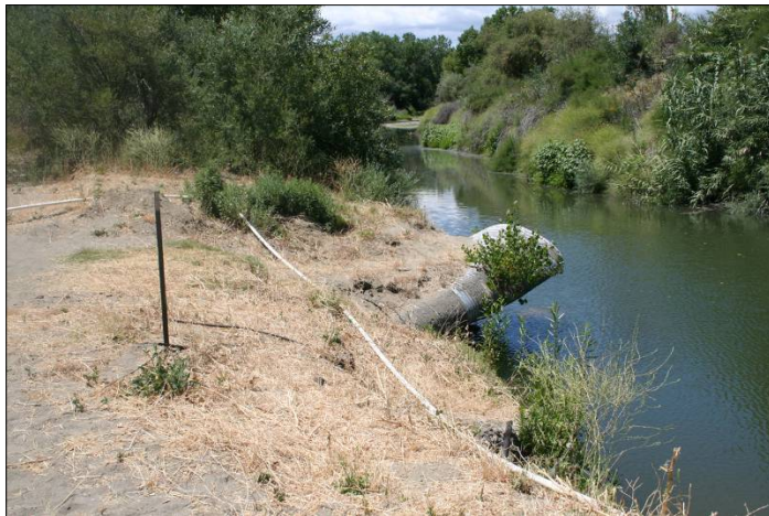
Figure 80. Drain pipe with unknown source.
