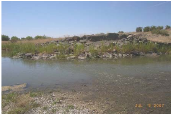
Figure 43: Erosion at upstream (south bank) spur dike, RM 21.3 in 2007 (left) and 2008 (right).
