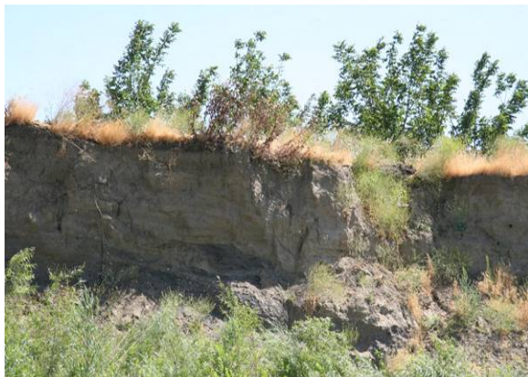
Figure 42: Active erosion at RM 21.6 north bank.
