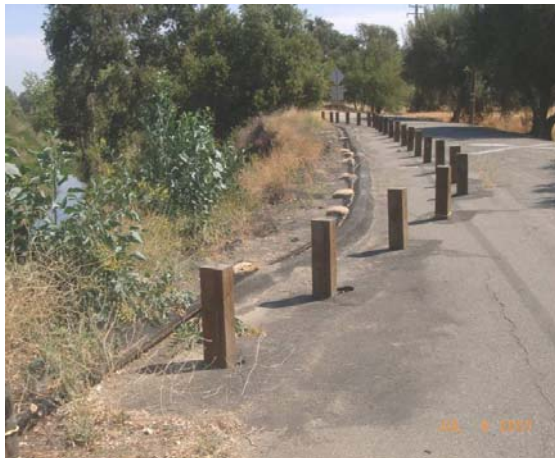
Figure 85. Huff's Corner CR-18 prior to bank stabilization work in 2007.
