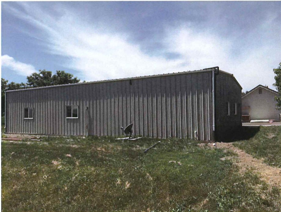
Photo Two Caption REAR VIEW (TAKEN 05/30/2019)
