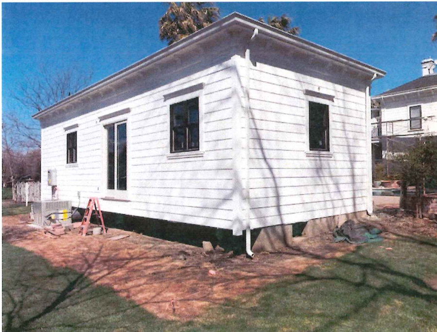
Photo Two Caption REAR VIEW (TAKEN 03/26/2018)
