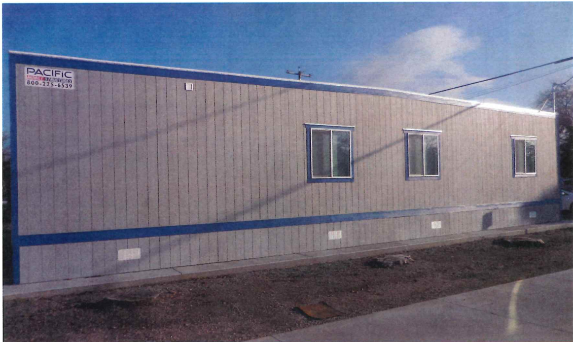
Photo Two Caption REAR VIEW (TAKEN 01/11/2018)
