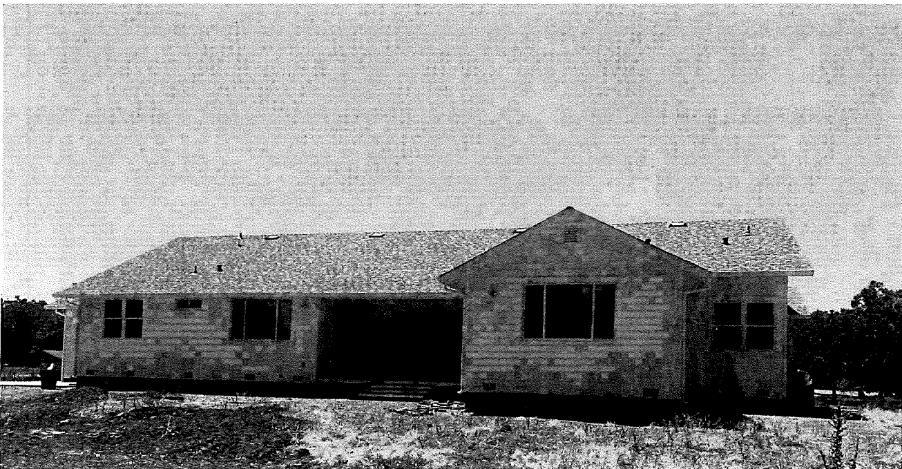
Photo Two Caption REAR VIEW (TAKEN 07/19/2019)
