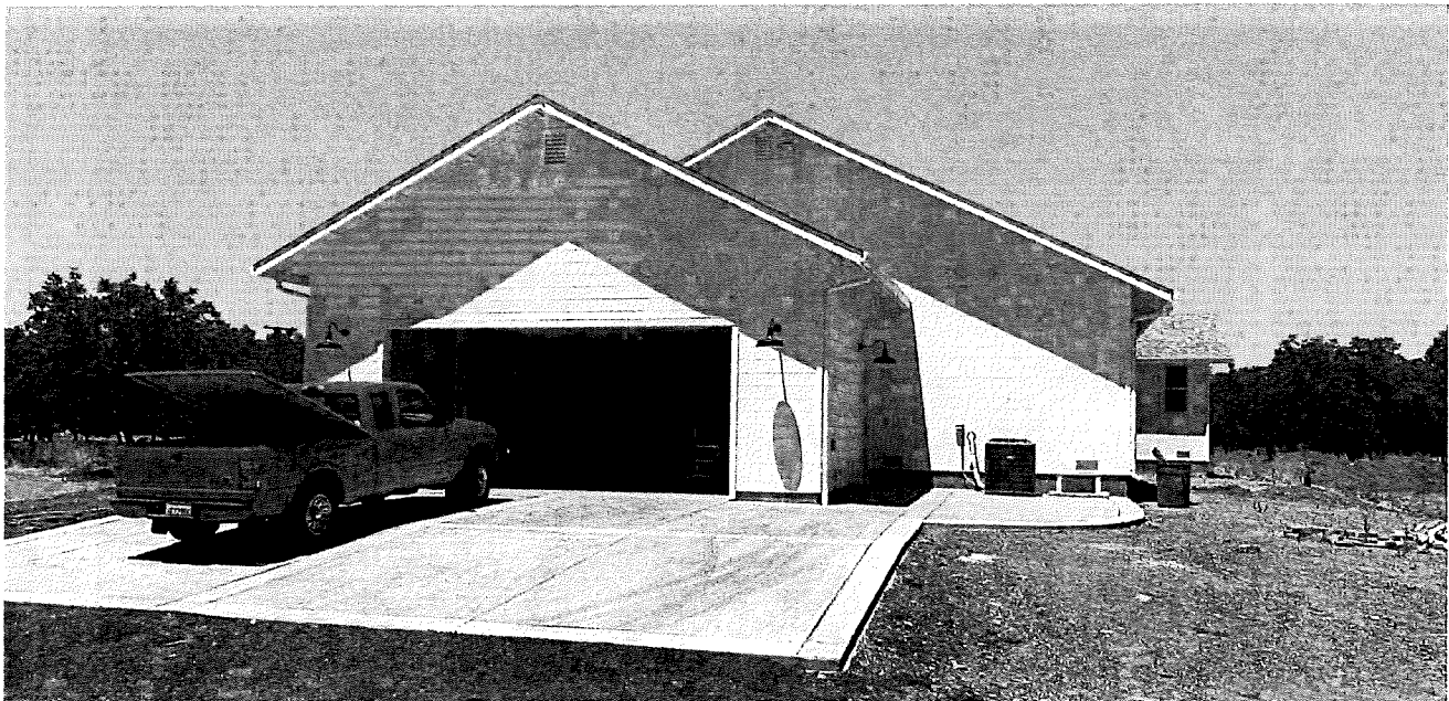
Photo Two Caption SOUTH SIDE VIEW (TAKEN 07/19/2019)
