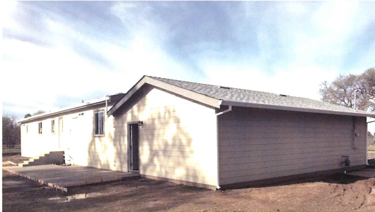
Photo Two Caption BACK OF MOBILE HOME (TAKEN 12/19/2018)
