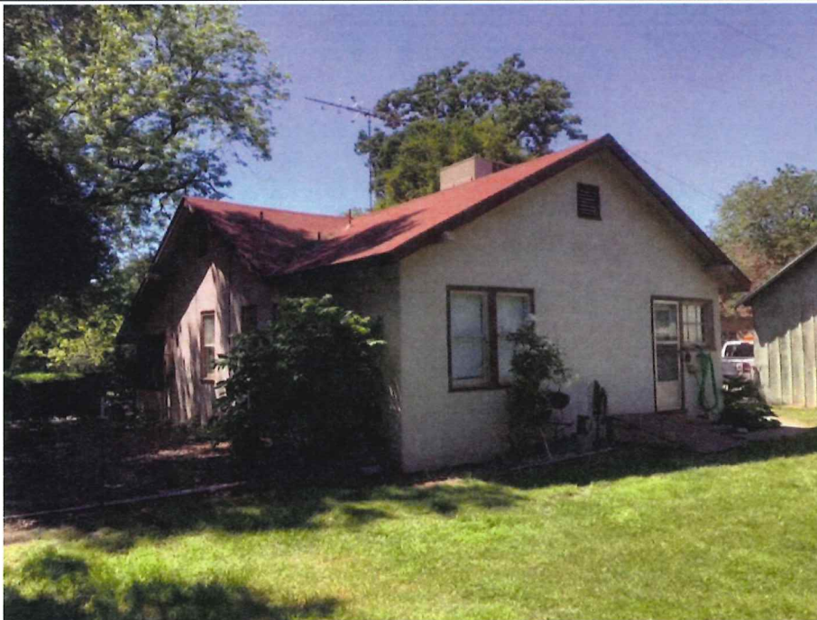
Photo Two Caption REAR VIEW (TAKEN 06/06/2017)
