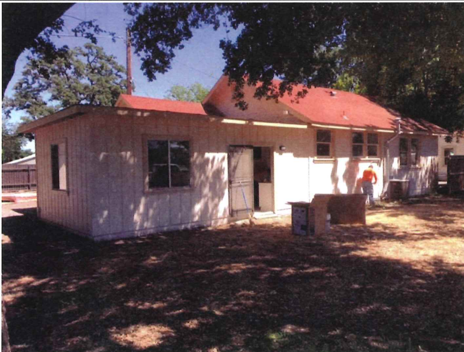
Photo Two Caption REAR VIEW (TAKEN 06/06/2017)
