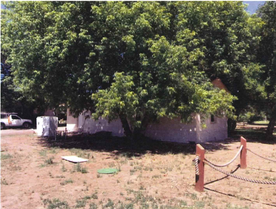
Photo Two Caption REAR VIEW (TAKEN 06/06/2017)
