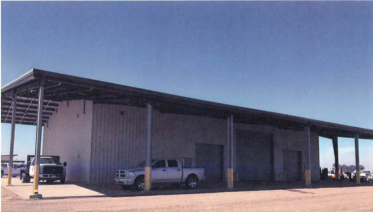
Photo One Caption EAST SIDE/LOOKING WEST (IMG_3715.JPG)
