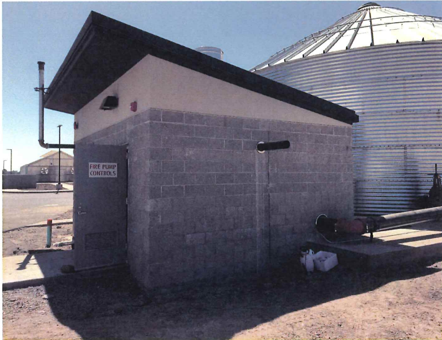
Photo One Caption NORTH SIDE/LOOKING SOUTH (IMG_3729.JPG)
