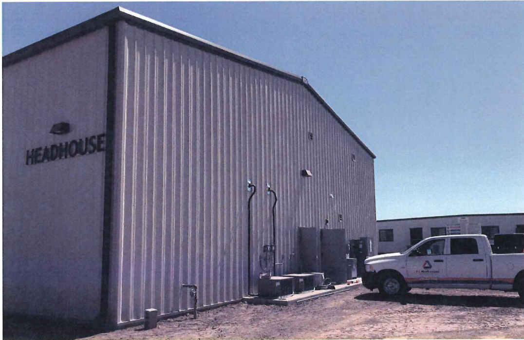
Photo One Caption WEST SIDE/LOOKING EAST (IMG_3734.JPG)
