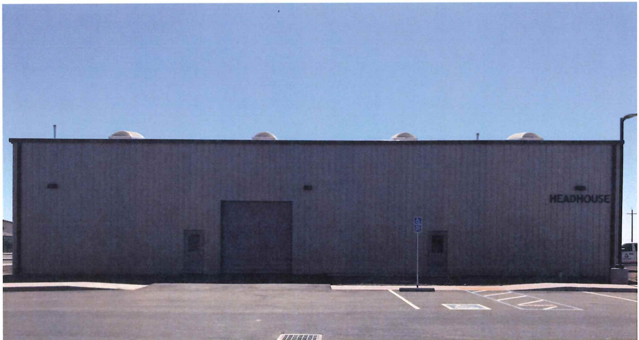
Photo Two Caption NORTH SIDE/LOOKING SOUTH (IMG_3733.JPG)
