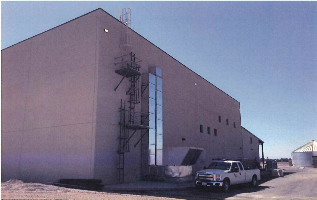
Photo One Caption NORTHEAST SIDE/LOOKING SOUTHWEST (IMG_3726.JPG)
