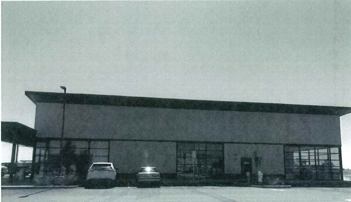
Photo One Caption NORTH SIDE/LOOKING SOUTH (IMG_3717.JPG)
