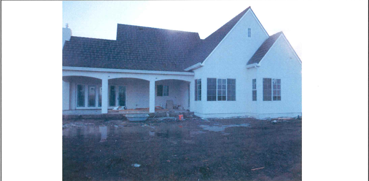
Photo Two Caption REAR VIEW (TAKEN 01/04/2018)
