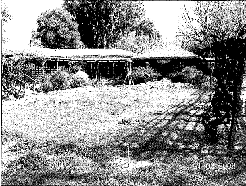
Front Looking Northeast
