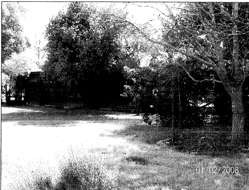
Rear Looking Southeast
