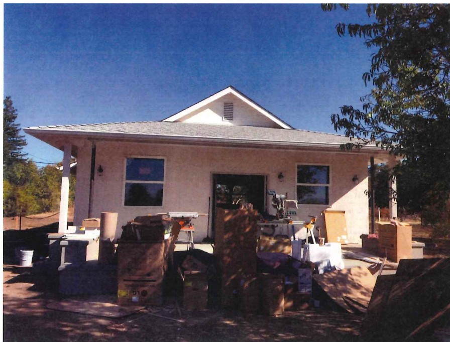
Photo Two Caption REAR VIEW (TAKEN 10/27/2017)
