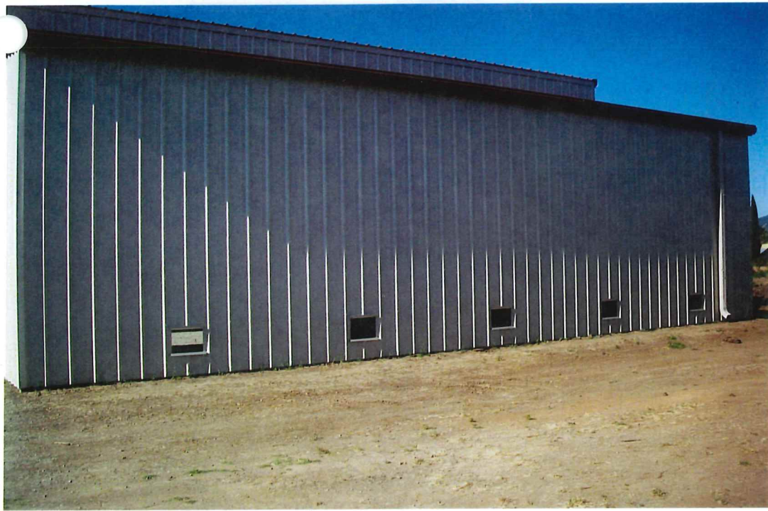
← 5 Flood vent North Face
