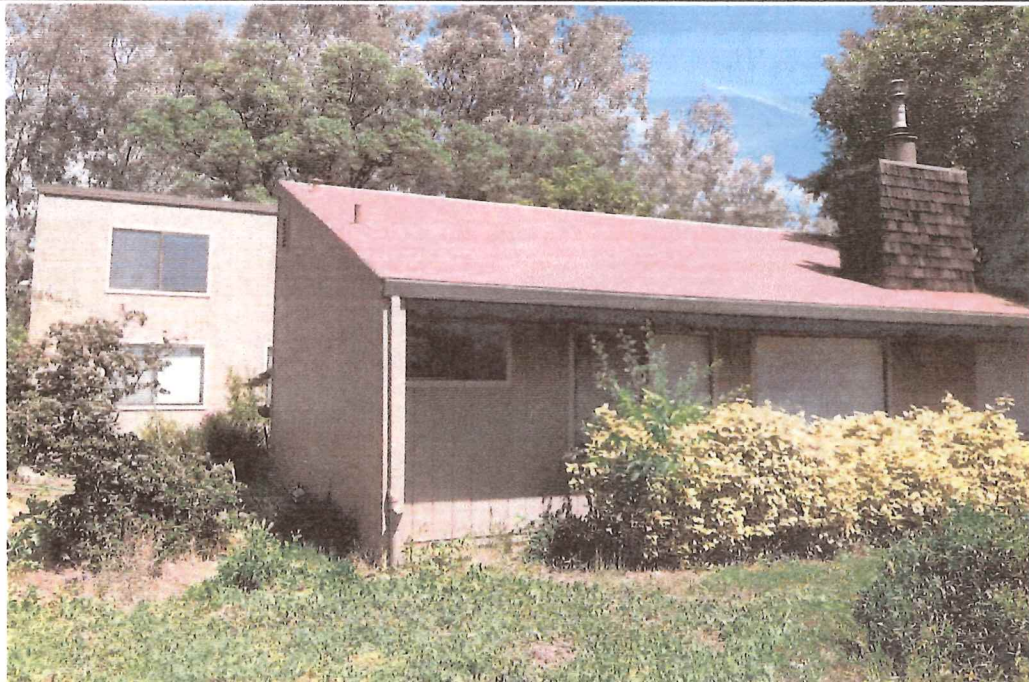
Photo Two Caption WEST SIDE VIEW (TAKEN 06/05/2019)
