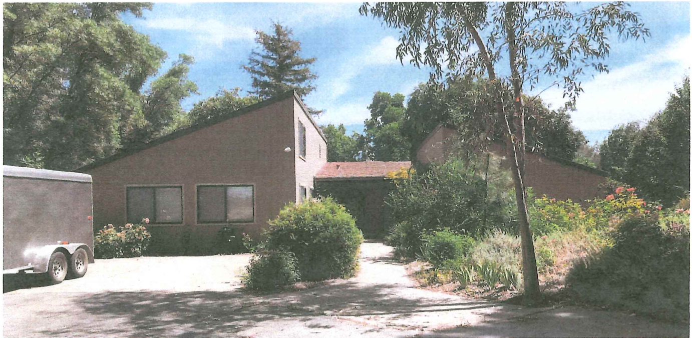
Photo One Caption NORTH SIDE VIEW (TAKEN 06/05/2019)
