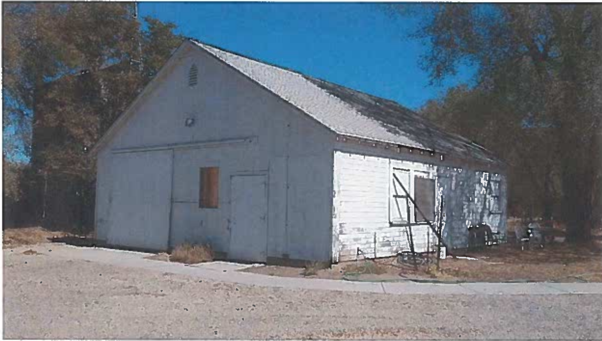
Photo One Caption Looking Northeast; Front and Right Sides
