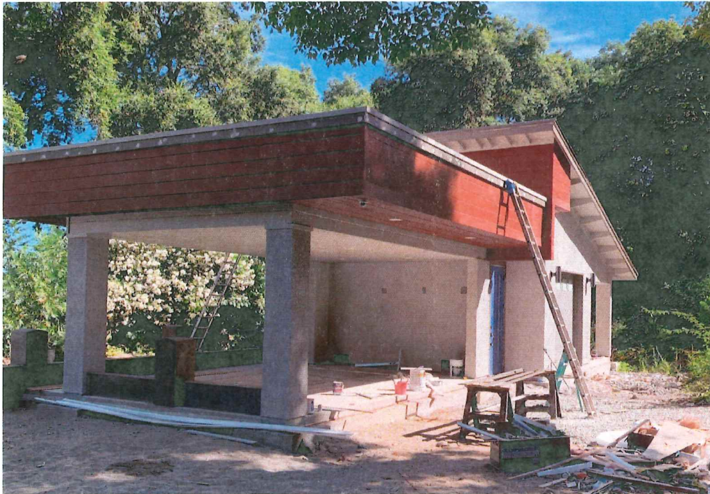
Photo One Caption SOUTH & WEST SIDE VIEWS (TAKEN 07/22/2019)
