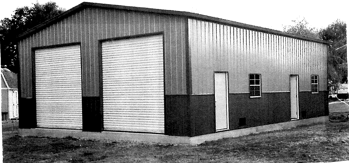
Photo Two Caption: LOOKING WESTERLY AT CONSTRUCTED BUILDING
