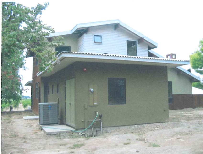
Rear View, Looking West – 08/06/2007
