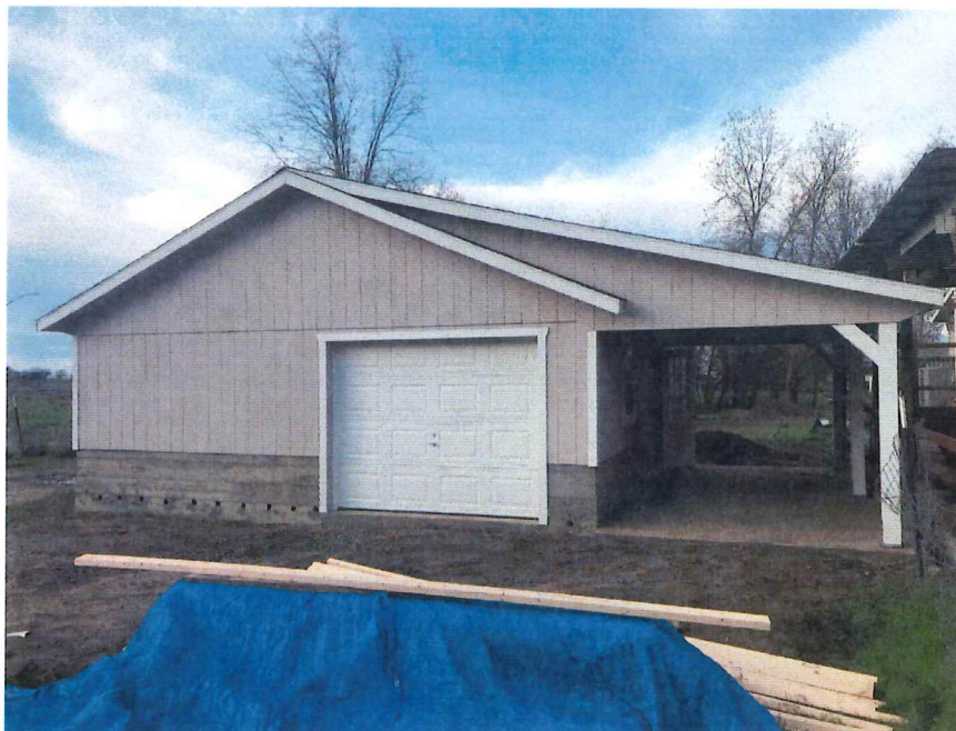
Photo Two Caption REAR VIEW (TAKEN 02/20/2019)
