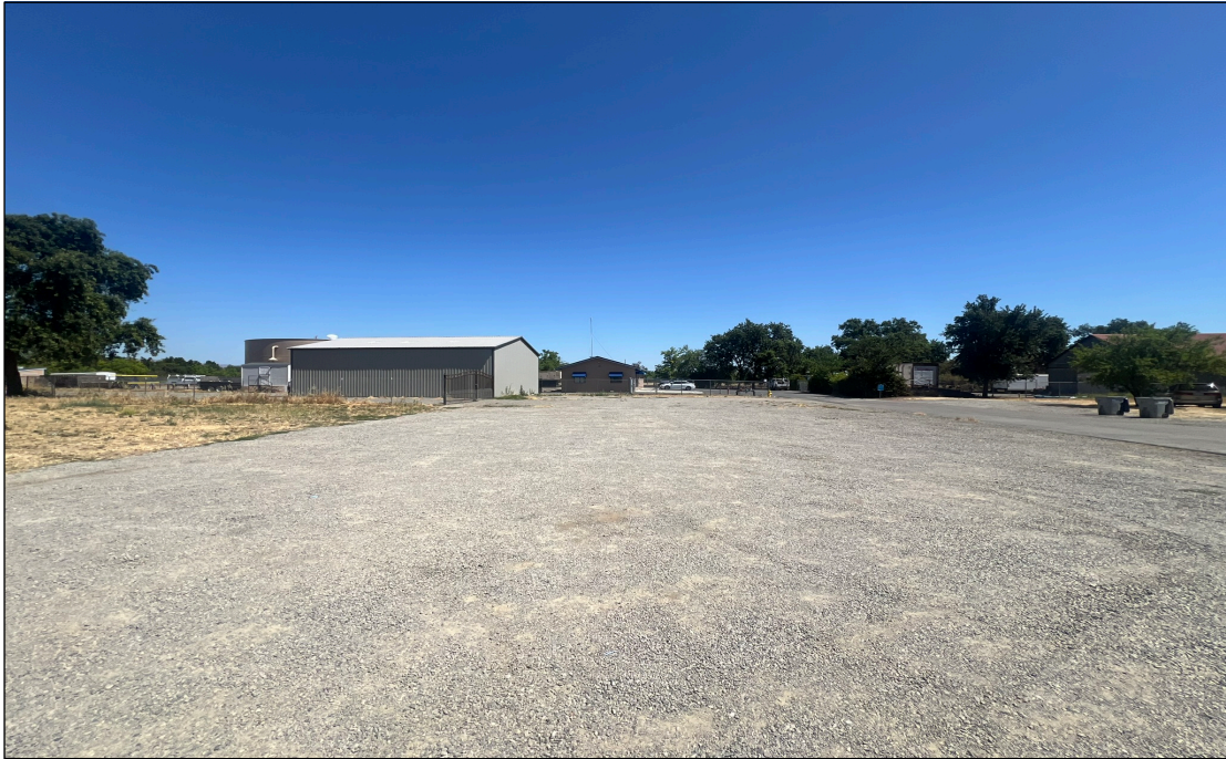
Existing view looking north from State Route 16
