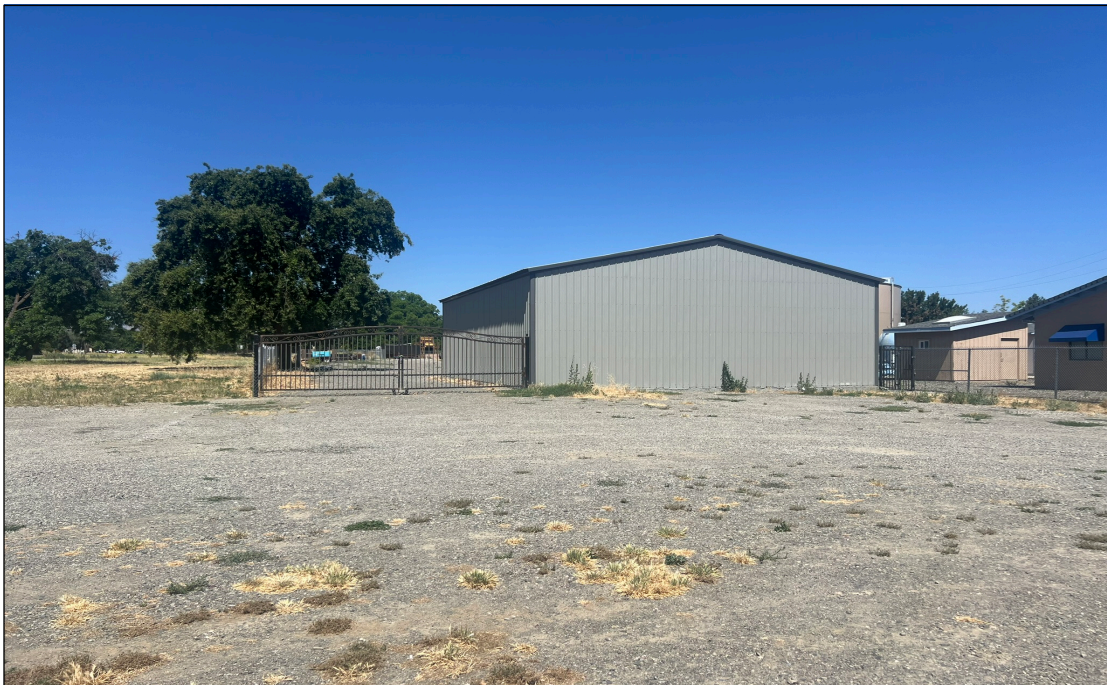
Existing view looking west at existing building
