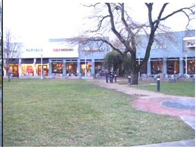
Figure 4: The pathway leading from this shopping center extends to a heavily trafficked street with additional commercial businesses. The path makes it easier for shoppers to walk to nearby businesses. The pathway is made of pervious material, allowing water to reabsorb into the water table.
