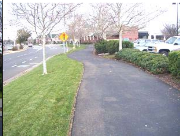
Figure 2: A wide buffer which includes a berm, bike/walk pathway, and landscaping can be used to conceal parking areas that abut a public right-of-way.
