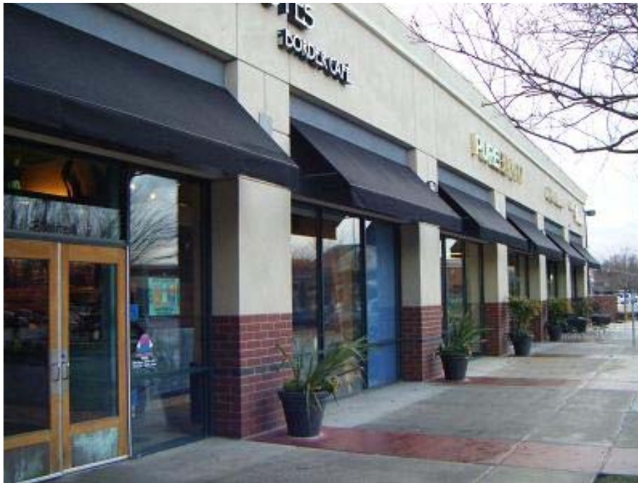
Figure 10: Large windows on this storefront provide an open and inviting feel. Pedestrian scaled design elements, such as planters and canopies, make the building pedestrian friendly.
