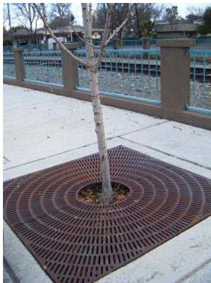
Figure 19: The grate at the base of this tree provides a walking surface, allows water to absorb into the roots, and can be replaced if the trunk of the tree becomes too large.
