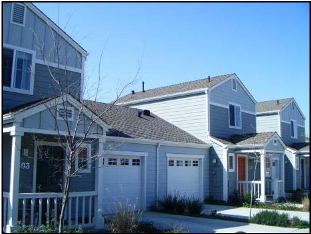
This example of compact development shows attached units with garages facing the main street. Note that the garages are recessed farther from the street than the porch.
