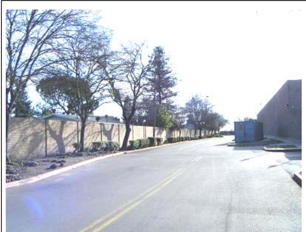
Figure 7: A masonry wall and a row of trees buffer the residential neighborhood from the industrial use. The loading docks and storage area are located away from the residential use.
